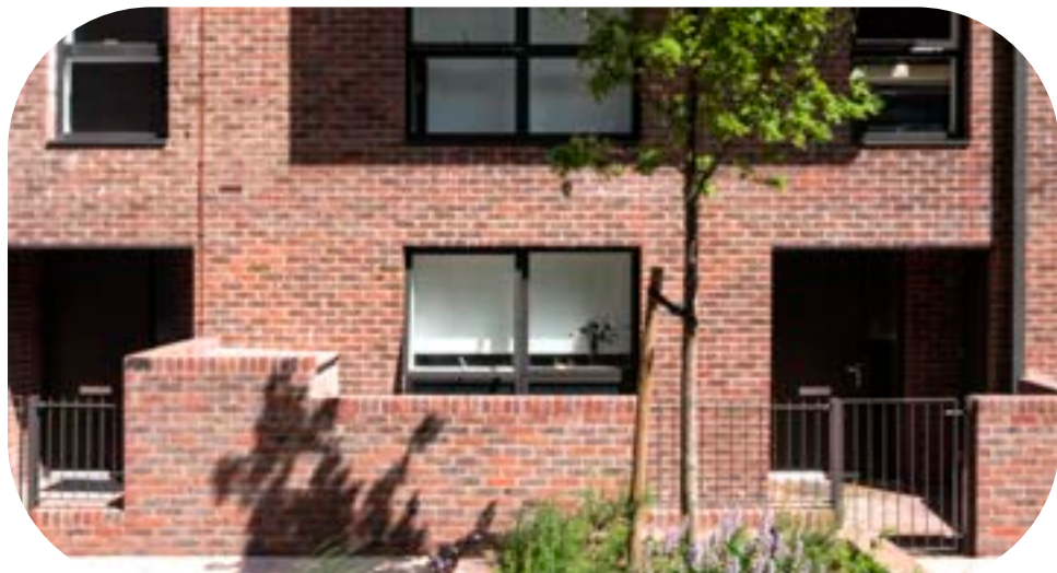
Brickwork colours and planted edge
