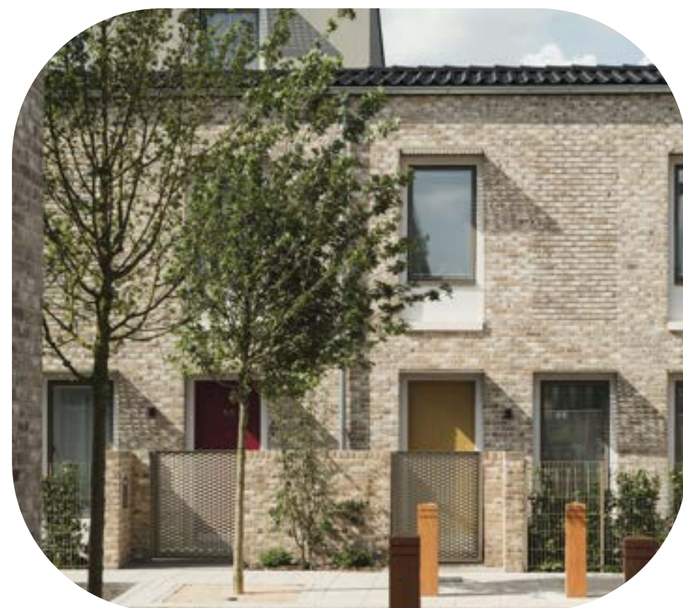
2 storey brick, on-street housing
