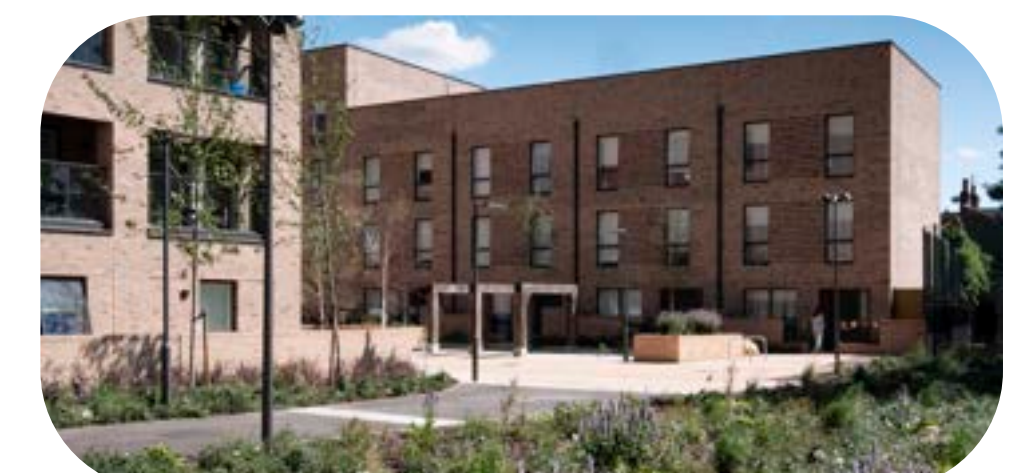
Three storey building with brickwork detail
