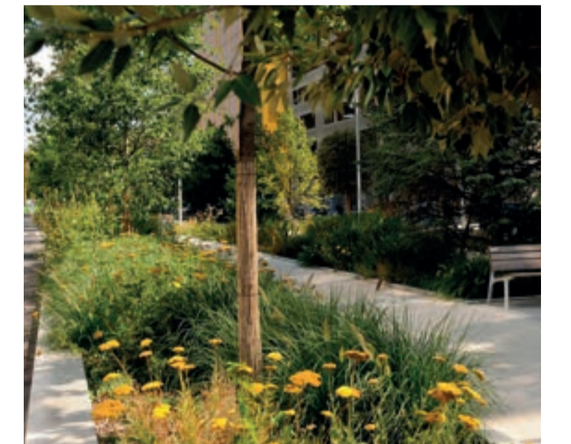
Planted Rain Gardens
