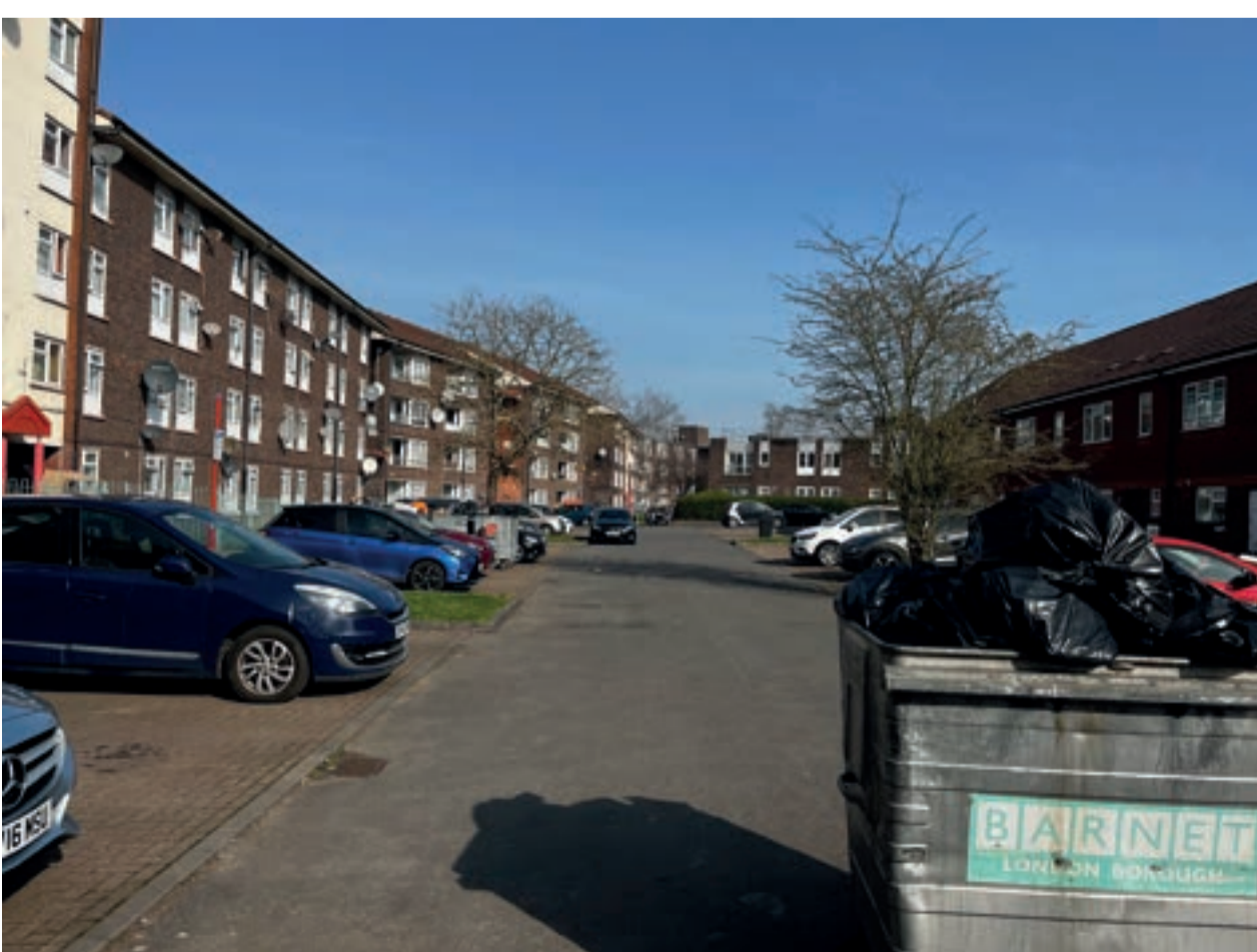
Existing parking courts
