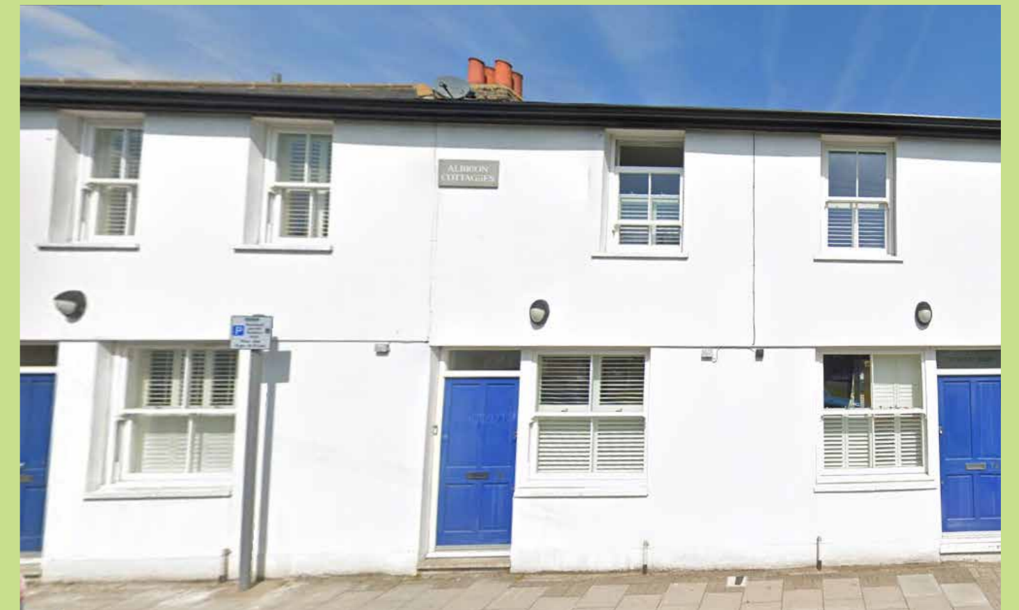
Albion Cottages, within the Wood Street Conservation Area
