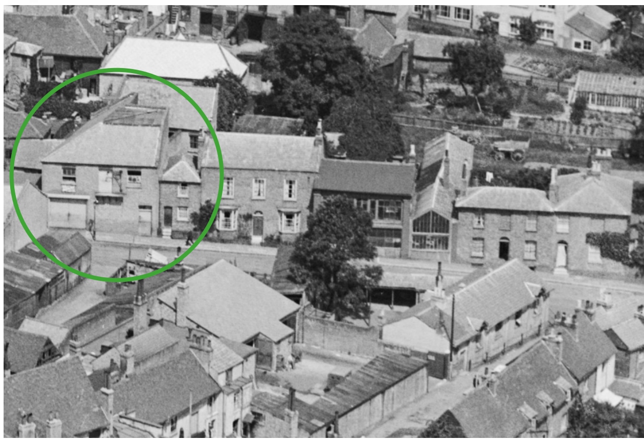
1928 Aerial Photograph showing existing brick building on site - proposed to be retained and refurbished (circled in green)
