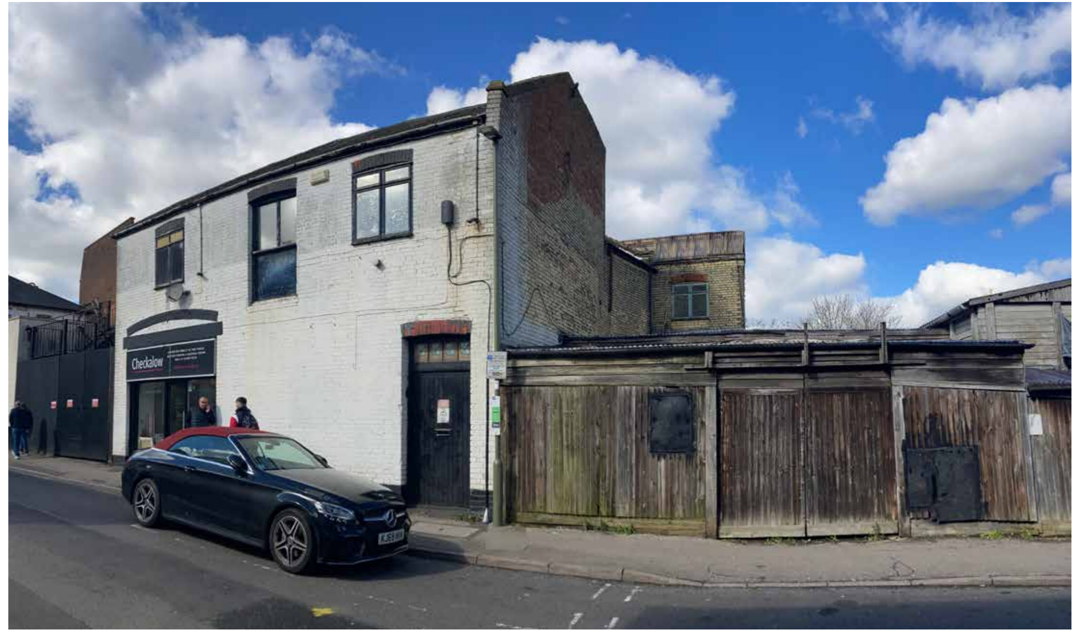
View 02 - View towards the existing brick building that we are working to retain and refurbish
