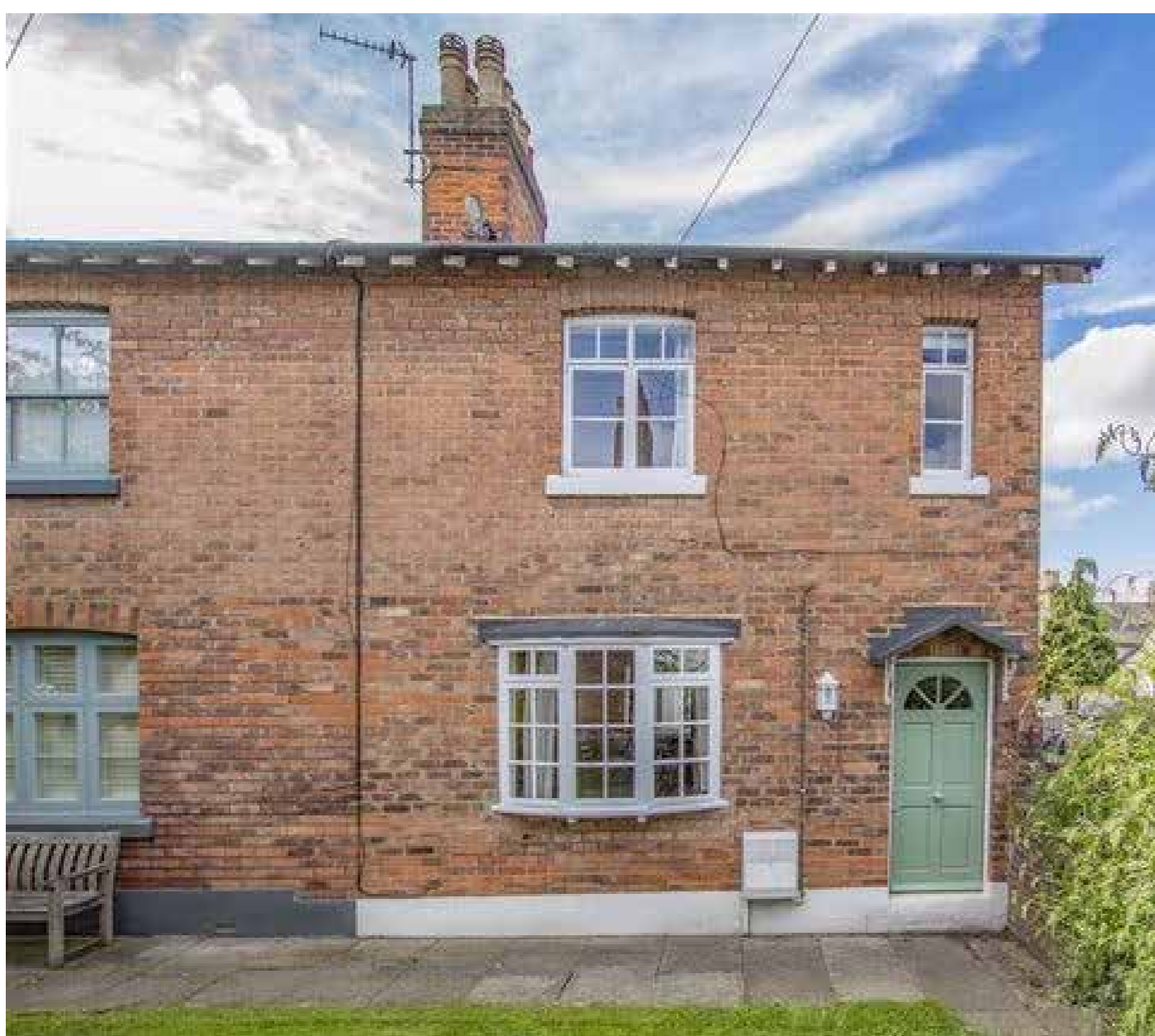
Midland Terrace, ordered and repeating elevations of the Railway Terraces, Cricklewood
