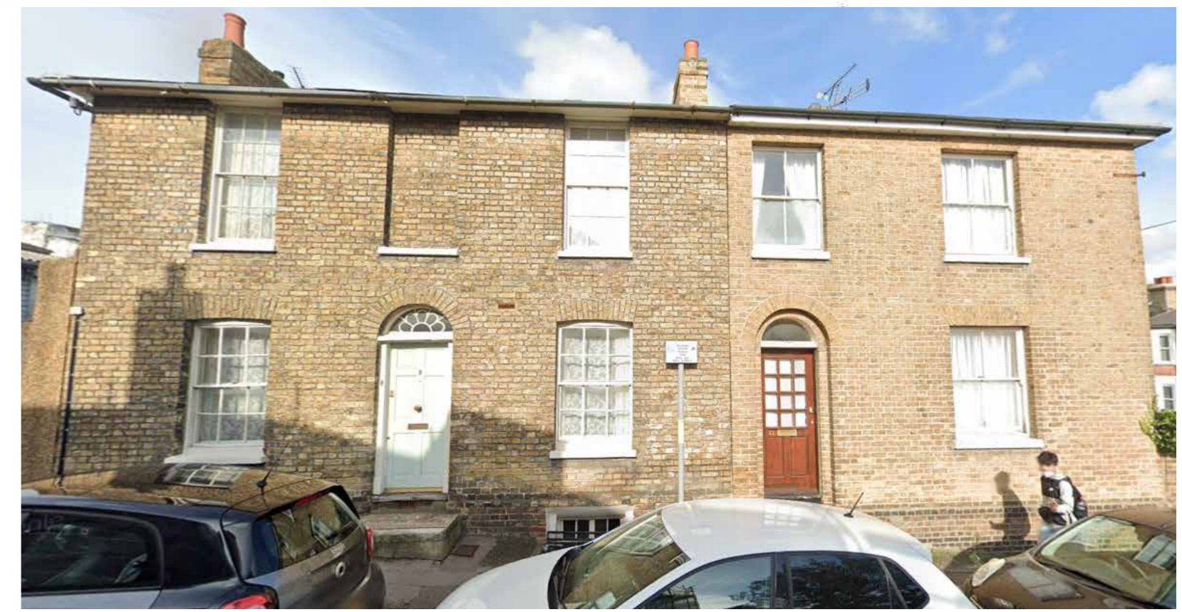
Front elevation of 9 & 11 Moxon Street
