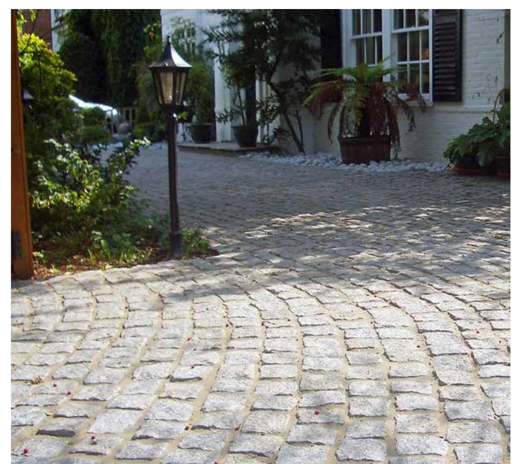
Cobbled paver and integrated flush planters
