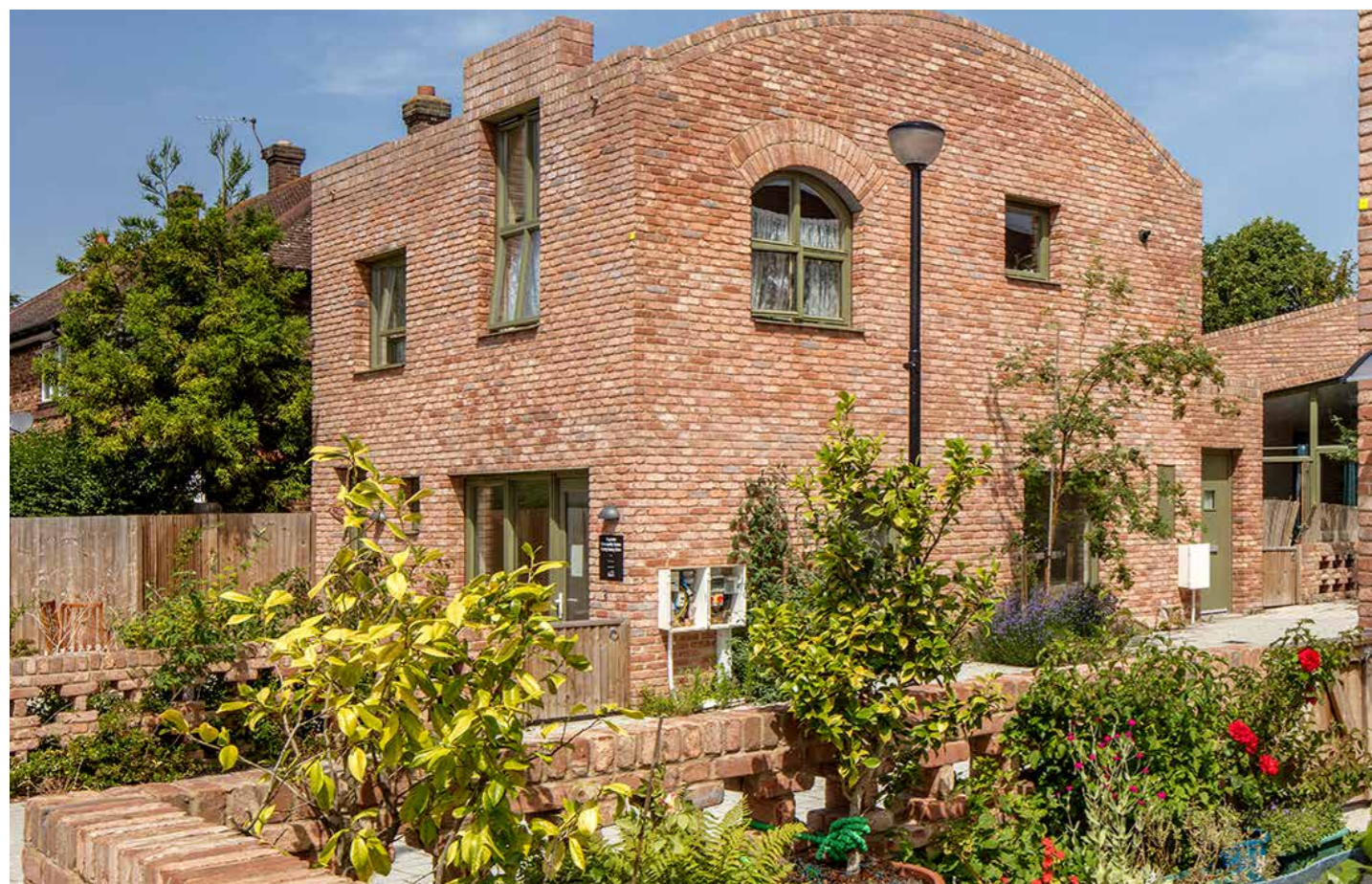
Brick details such as arched window heads and brick on edge parapets
