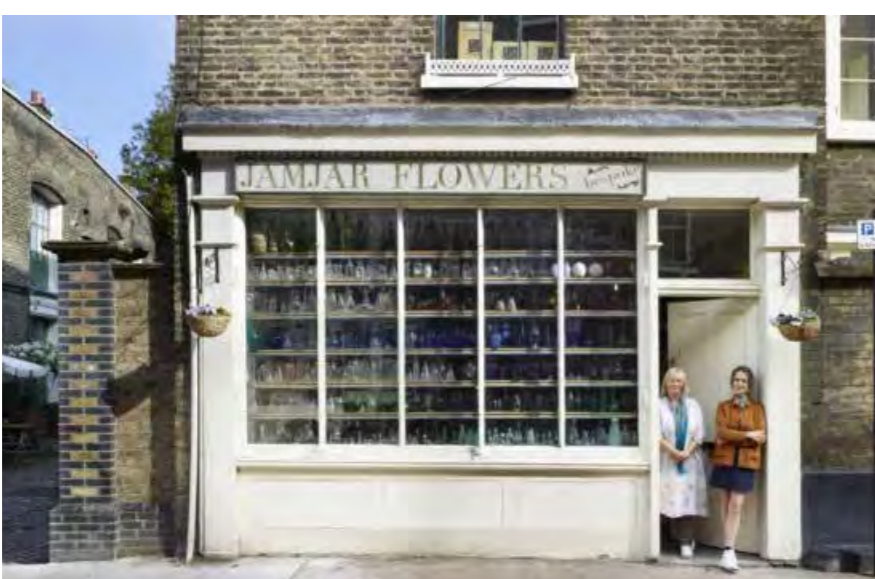
Precedent image of high quality traditional shop front with stallriser, glazing bars etc
