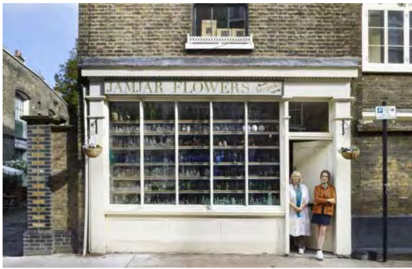
Precedent image of high quality traditional shop front with stallriser, glazing bars and timber surround
