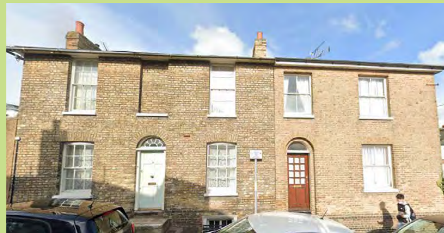
9 & 11 Moxon Street - local heritage assets adjacent to the site. 9 Moxon Street (left hand side) is a beautiful Grade II listed house
