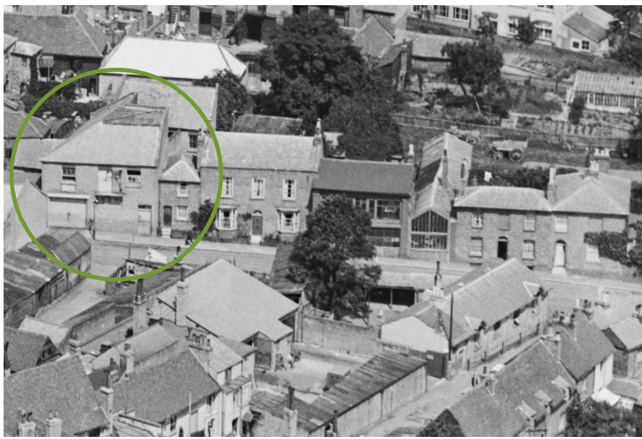
1928 Aerial Photograph showing existing brick building on site - proposed to be retained and refurbished (circled in green)
