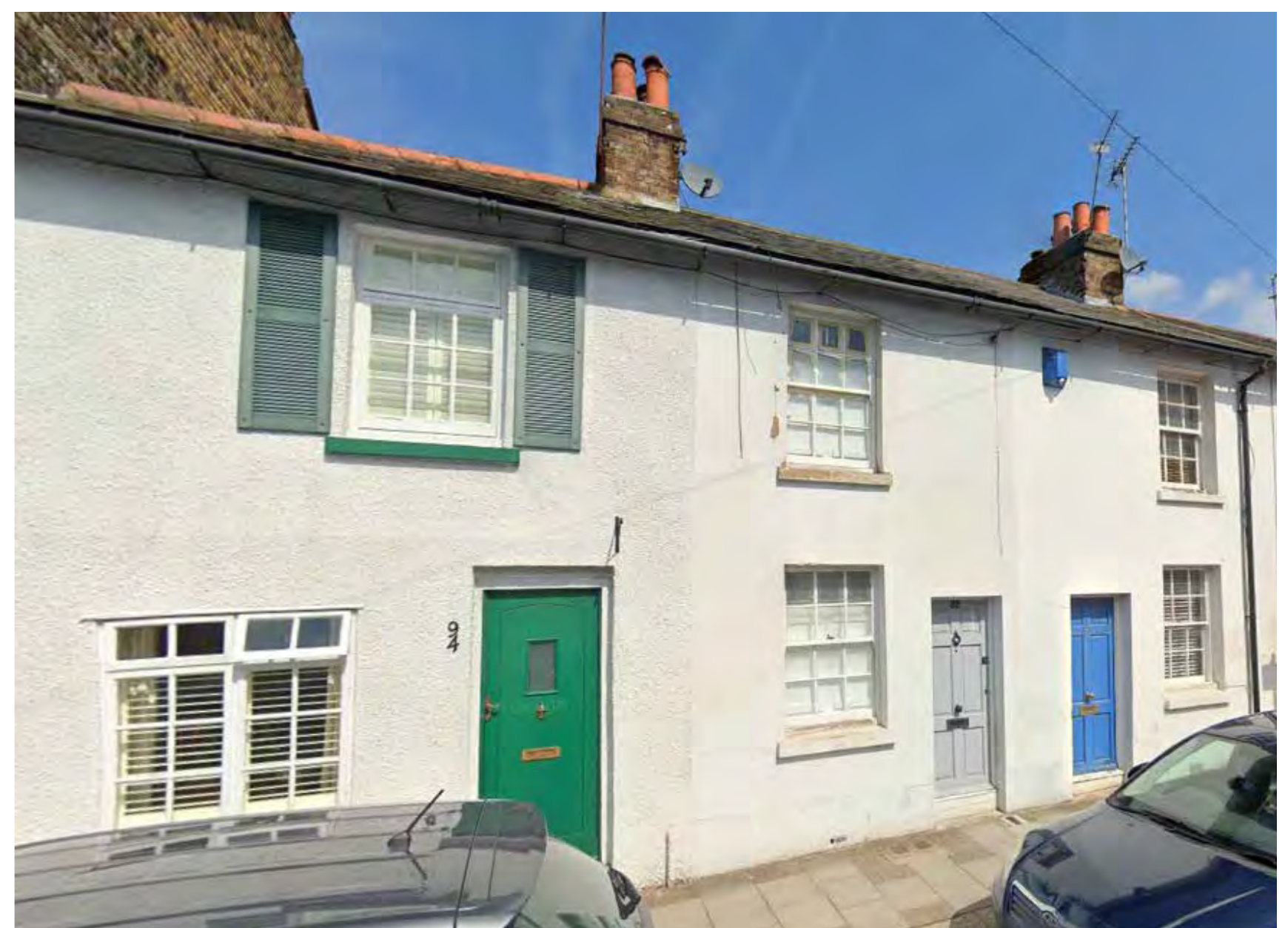
Albion Cottages, within the Wood Street Conservation Area
