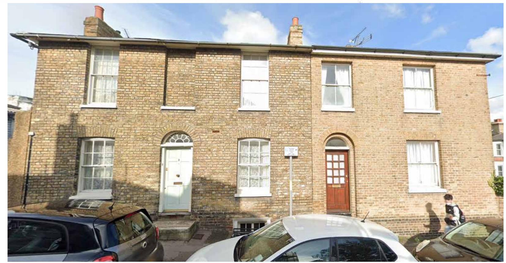
Front elevation of 9 & 11 Moxon Street
