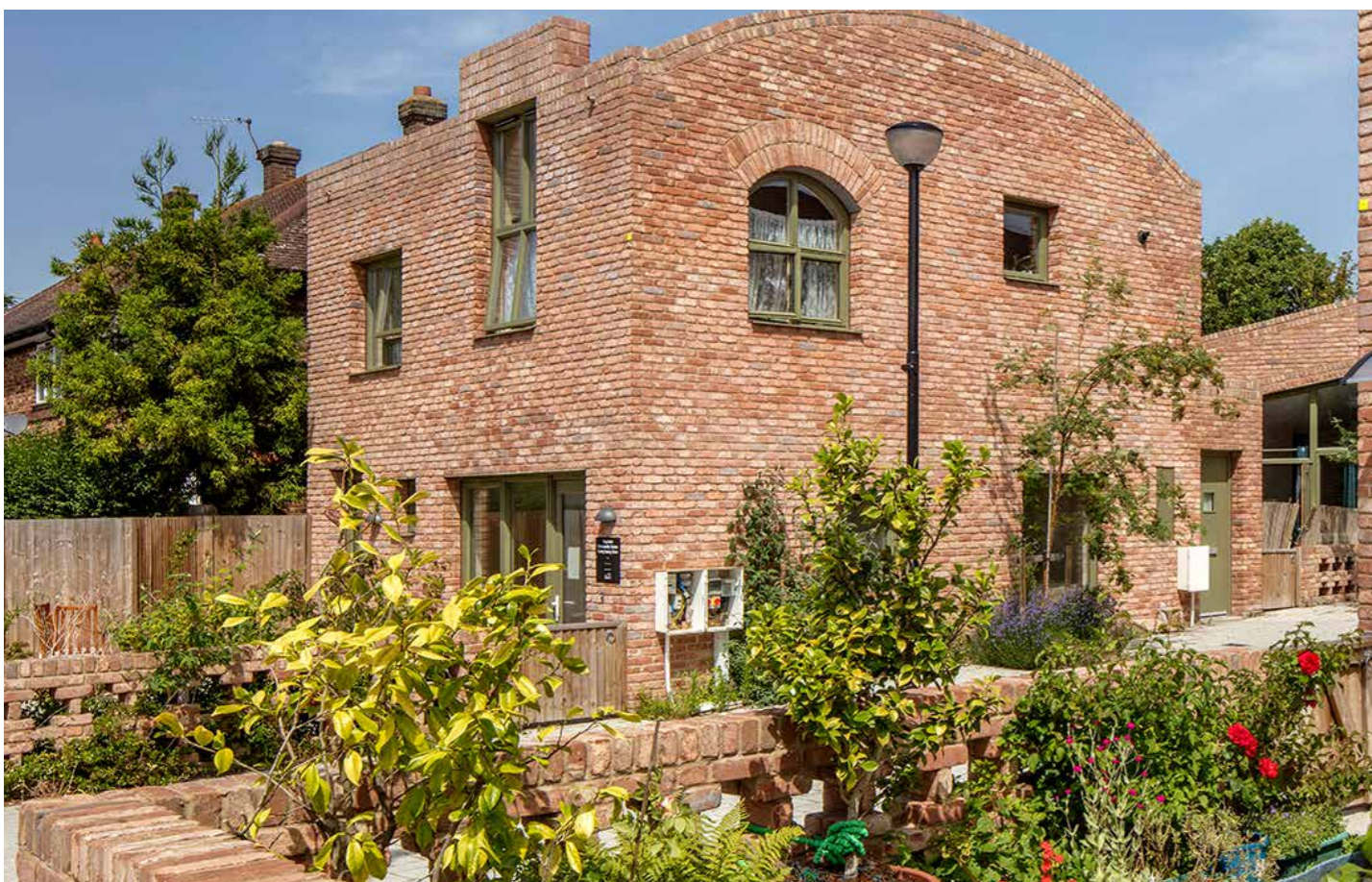
Brick details such as arched window heads and brick on edge parapets
