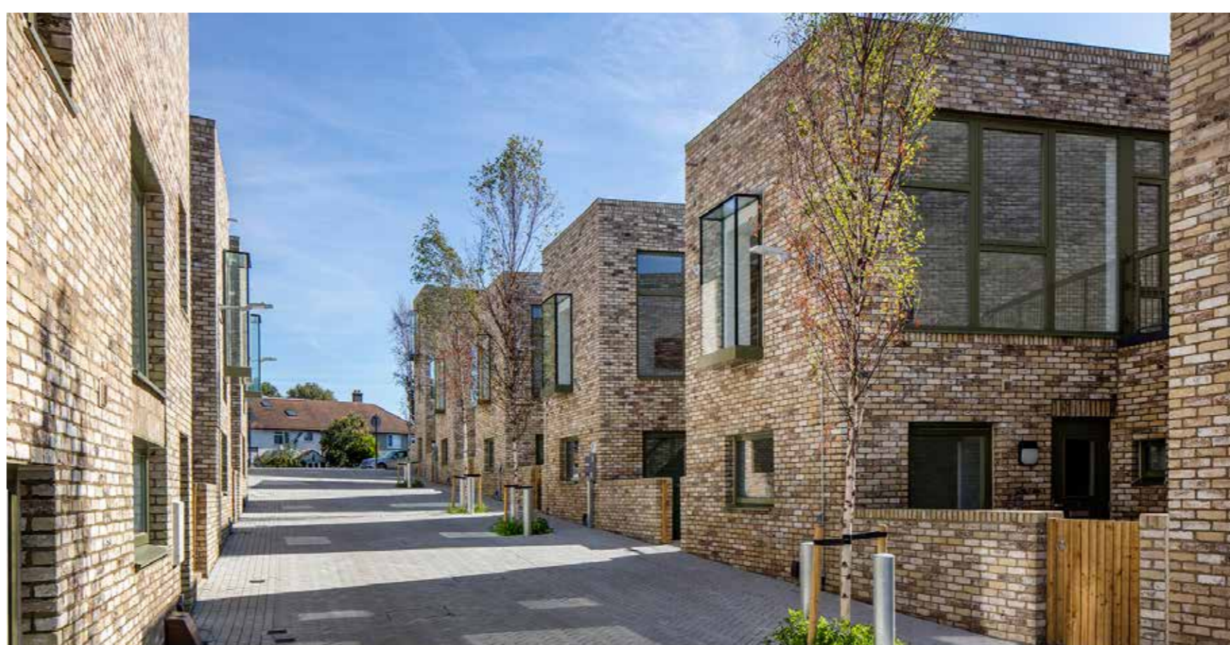
Shared surface mews street
