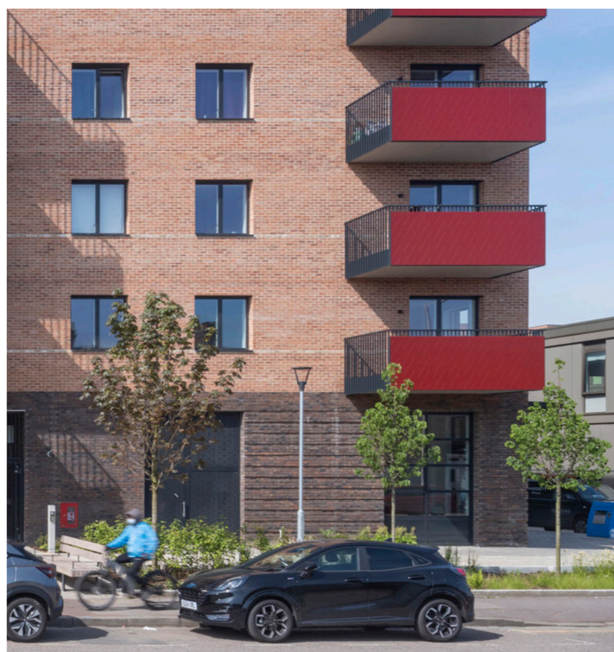
▲ Fig 7. Gascoigne East Phase 3a
